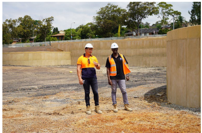
Earthworks are finished and walls are in place – landscaping next (March 2022)
