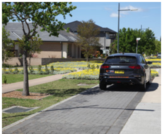
Kerbless areas for passive irrigation with inlet pits at Moorebank. Image - (ASPECT Studios)
