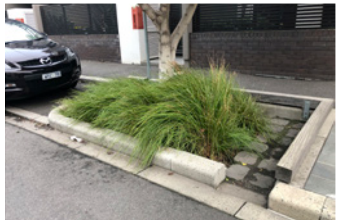
Raingarden with a slotted kerb in lieu of car parking, Rozelle. Image - (ASPECT Studios)
