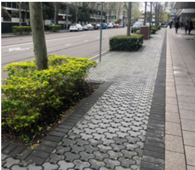
Permeable paving for street trees on Rider Boulevard, Rhodes. Image - (ASPECT Studios)
