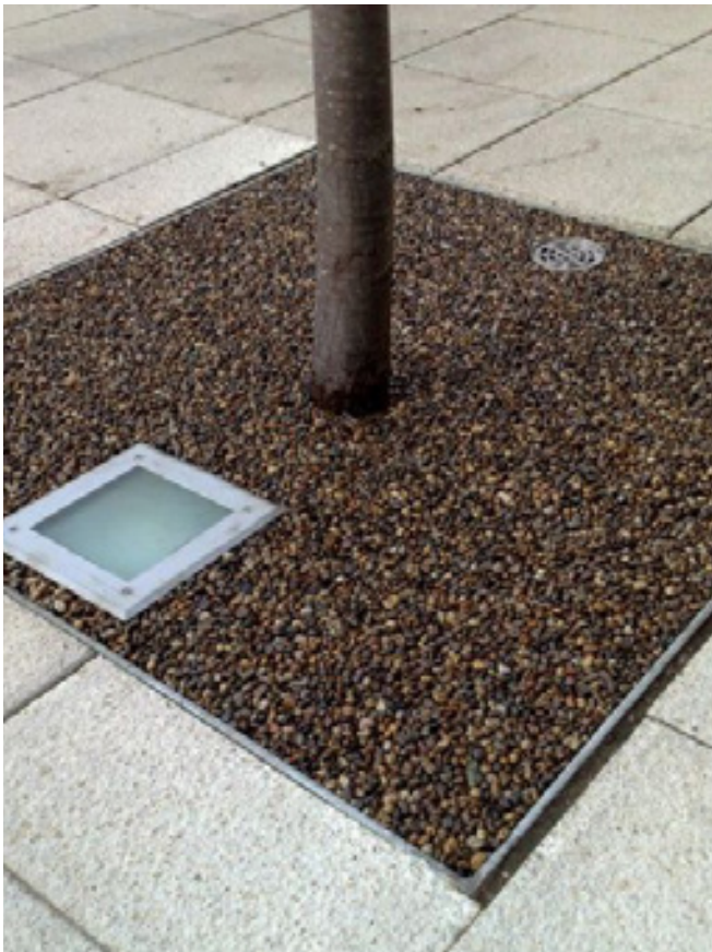
Tree pit Terrabond Image - (Resin Drives)
