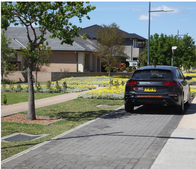
Kerbless areas for passive irrigation with inlet pits at Moorebank (source: ASPECT Studios)
