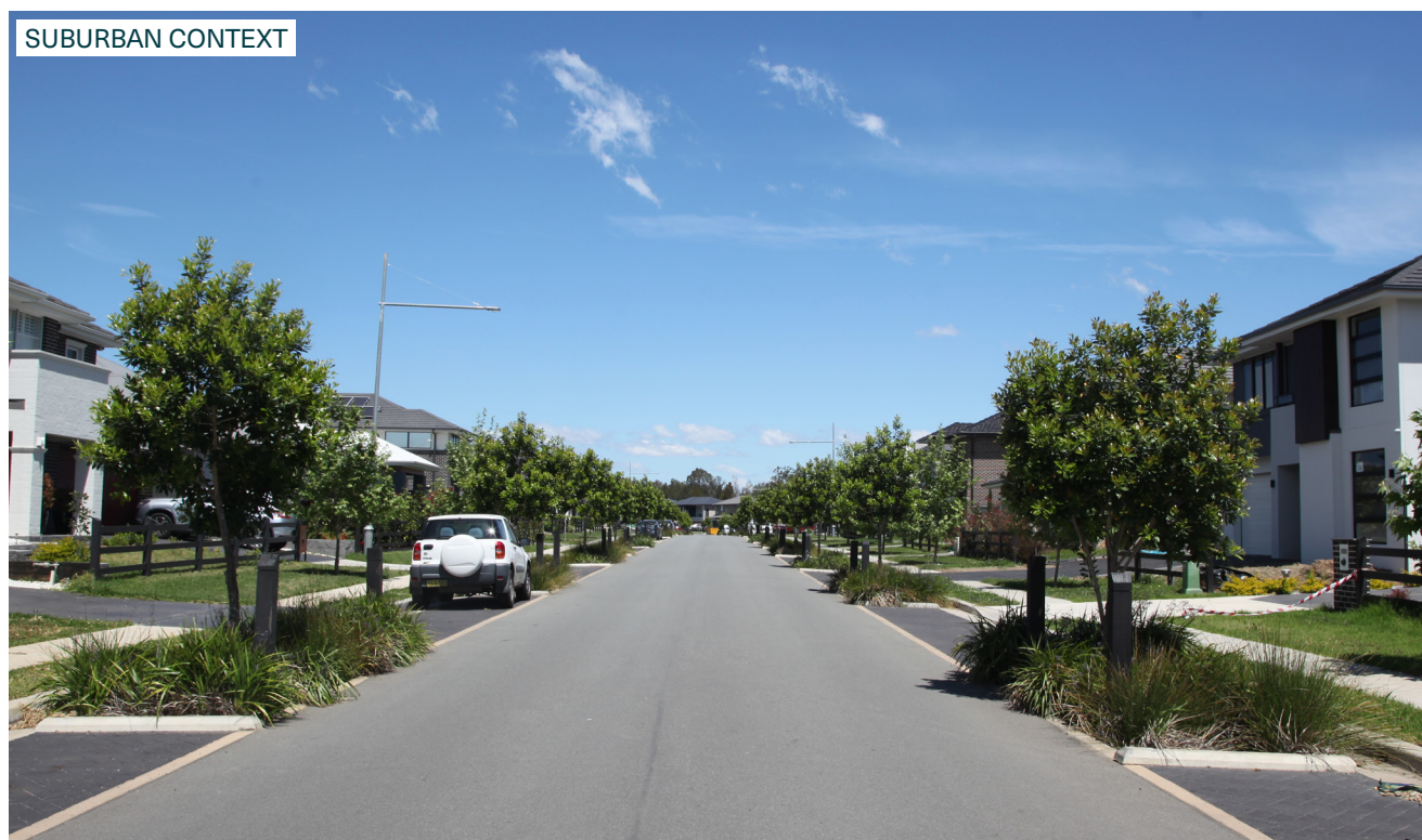
Precedent: Pennyroyal Boulevard, Denham Court (source: Google)
