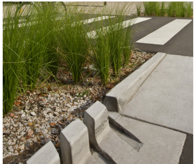
Slotted kerb for passive irrigation on Bourke Street, Surry Hills (source: Simon Wood)
