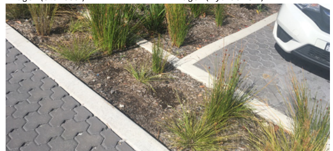
Permeable car park paving. Image - (ASPECT Studios)
