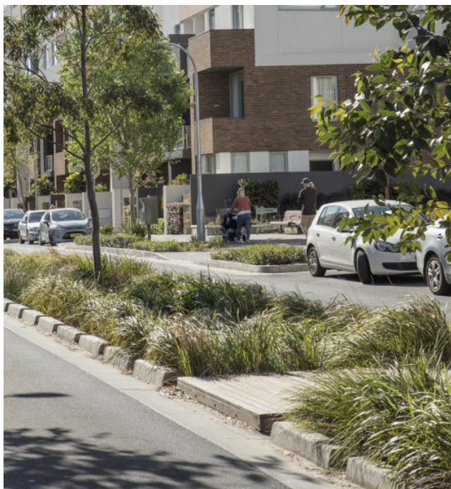
Kerb cuts for passive irrigation in Harold Park. (credit: ASPECT Studios and Simon Wood)
