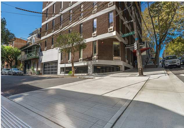
Continuous footpath allow for safer pedestrian travel on Foveaux Street, Sydney. (credit: City of Sydney)
