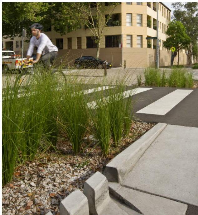
Kerb cuts for passive irrigation on Bourke Street, Surry Hills. (credit: City of Sydney and Simon Wood)
