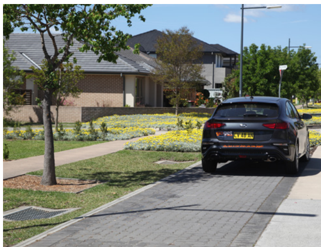
Kerbless areas for passive irrigation with inlet pits at Moorebank. (credit: ASPECT Studios)
