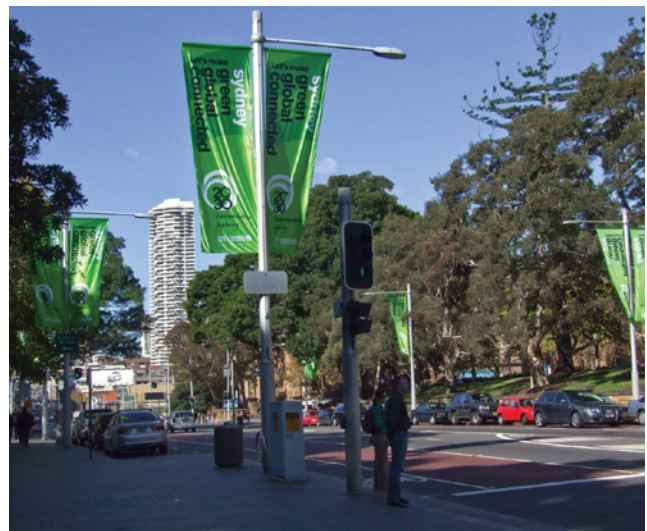
Multi-function poles can combine services infrastructure with banners. Image - (Hub Group)
