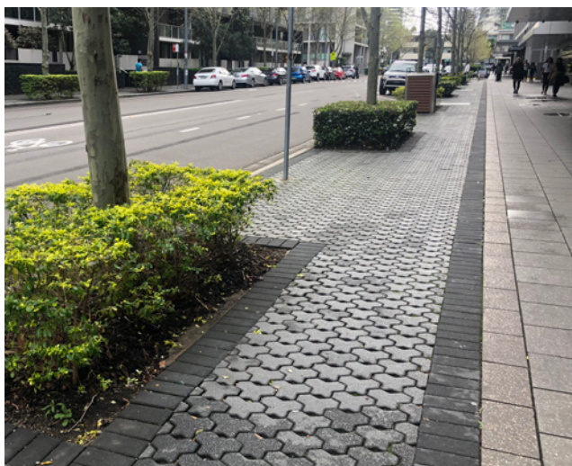
Permeable paving for street trees on Rider Boulevard, Rhodes (credit: ASPECT Studios)
