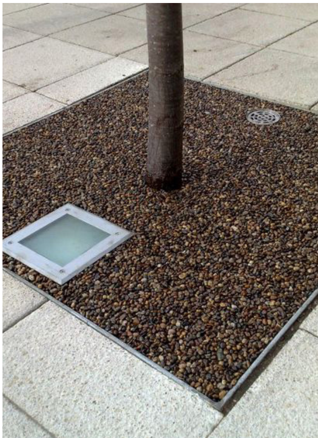
Terrabond tree pit (credit: Resin Drives)
